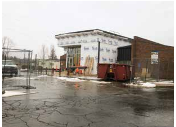
Exterior of the Vienna branch during construction.
